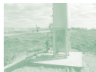
In April 2004, installation works started on gas pumping station and flare in the current landfill 'Skede'.
