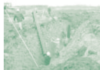
Construction works start in spring 2004 with the main pipe-lying at the Grobina Poligons which is the new regional sanitary landfill with energy cell technology for biodegradable waste.
