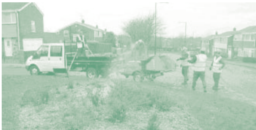
The decision to chip all appropriate arboreal waste on site reduced fuel consumption and lost time, and also made financial savings of approx. £1000 per week in City Grounds which is a unit within Environmental Services.
