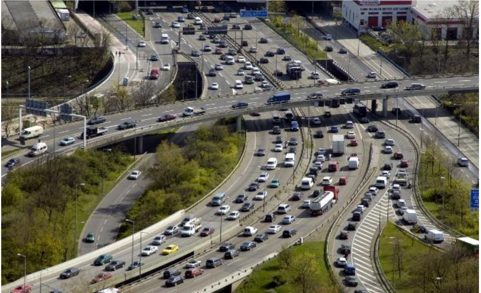
City motorway, Berlin (Germany)
